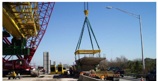
Twin Path® Slings can be cost effectively repaired, if the core fibres are not already cut or damaged.
